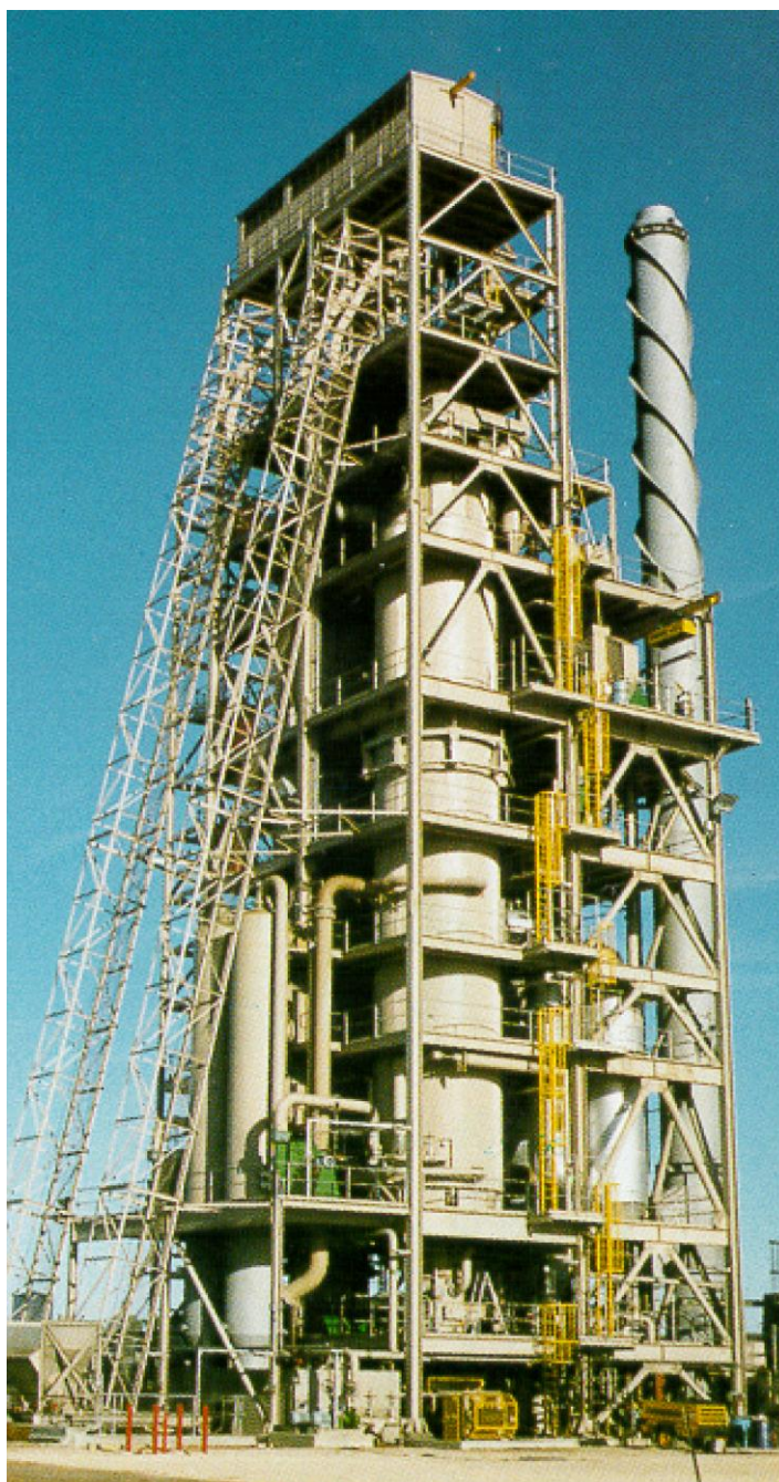
Figure 9 Lurgi shaft charcoal kilns at Simcoa
