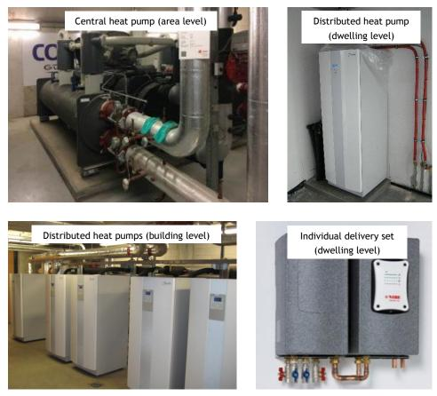
Figure 12 - Examples of central and distributed heat pumps (dwelling and block level) and connection set
