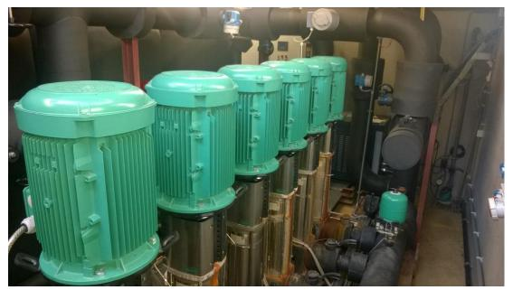
Figure 35 - Battery of pumps in an underground Minewater pumping station
