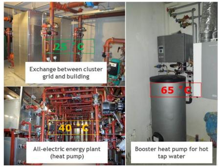
Figure 29 - Elements of the energy plant in a large (utility) building
