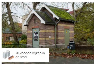
MS-MS station (3-23kV)
