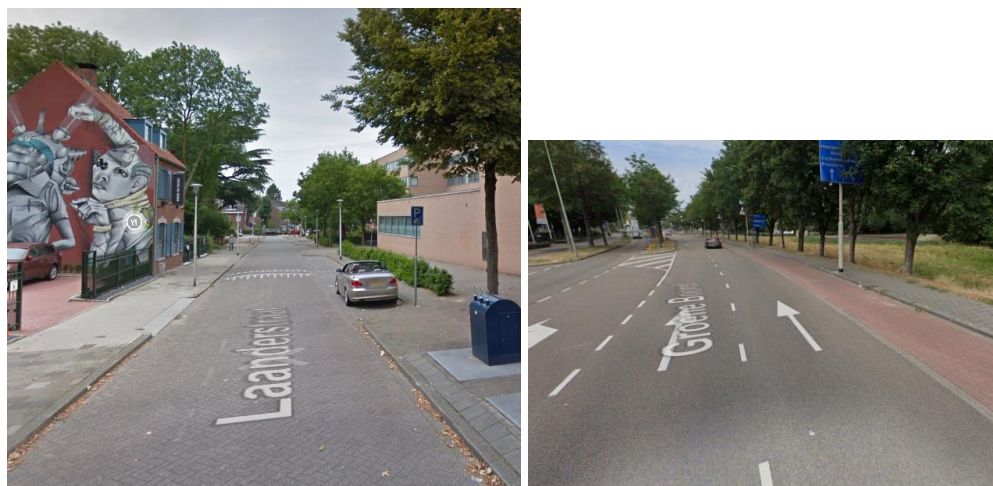
Figure 15 - Two types of road surface: removable pavement (on the left) and asphalt (on the right)
