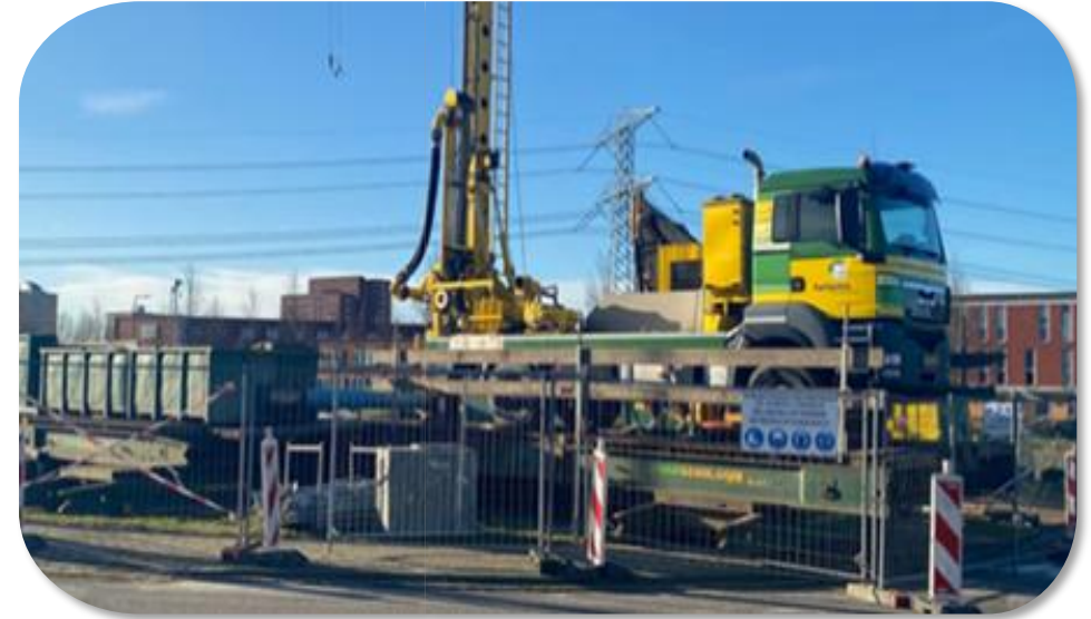
Boven: Proefboring Nesselande (IF Technology, 2020).
